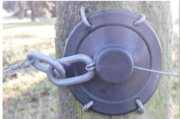
Zoom of circled feature (adjacent photo). The Isolator and Link set-up take on the fence strain when the gate is opened.
