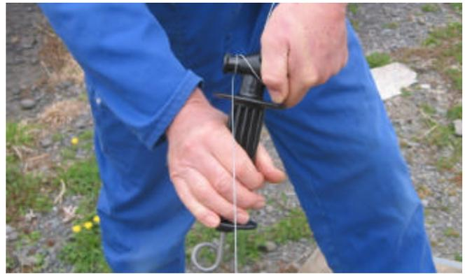
Step 8: Wind around the small drum at least three times to ensure contact and therefore conductivity with the exposed metal strip. The small drum is also useful as a fine tension adjuster.
